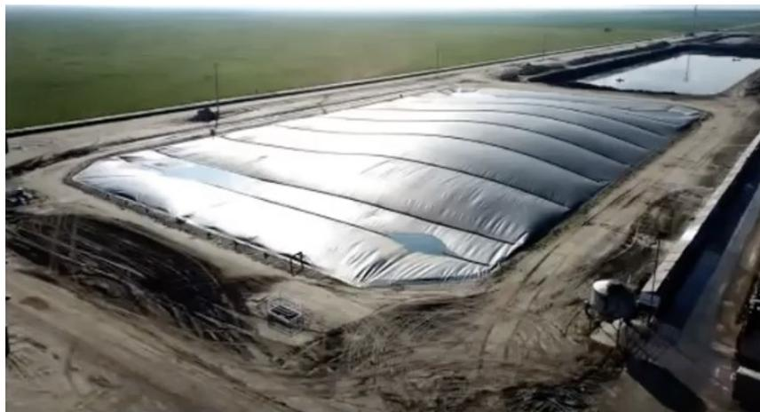
Pictured above is an in-ground digester; one of few different designs of anaerobic digesters (AD). The digester cover is inflated, which means there is gas buildup underneath. The gas built up is biogas. In-ground digesters look a lot like a lagoon, but the two are designed and managed differently.
